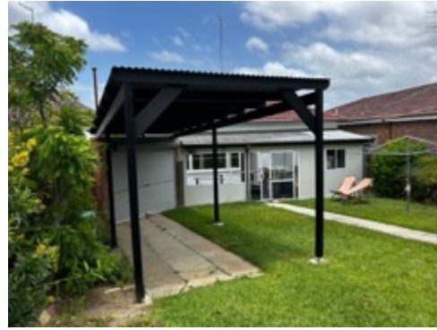
Source: SWAD PL Photograph 2: Existing Rear Façade
